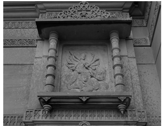
Figure 16. CNC carved external stone panel prepared on the basis of a clay model.
